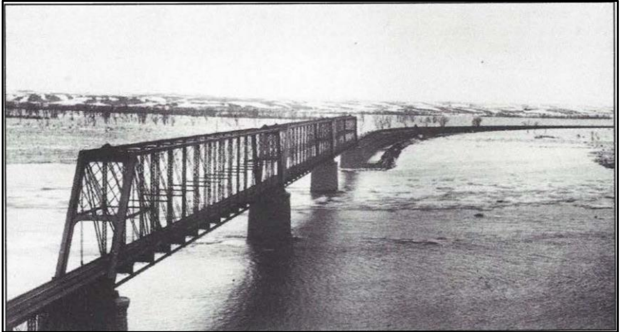
Figure 17: Missouri River Flooding in 1887 Inundating All Four Historic Bridge Piers (Murphy 1995).
