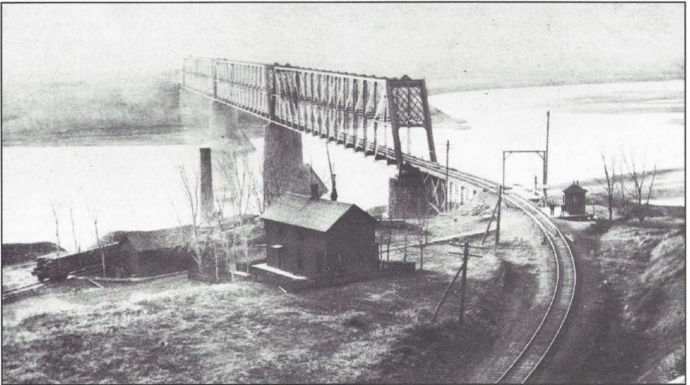
The Northern Pacific Railway Company posted a watchman at the east end of the bridge from its completion in 1883 until the replacement of its spans in 1905. The watchman's shack is on the right side of the track and his house is on the left side. Below the house are a toolshed and the pumphouse for the Bismarck Water Company. As designed by Morison, the tracks took a sharp turn before entering the east side of the bridge. In 1951 the Northern Pacific reduced the curvature in this area by making a deep cut into the hillside east of the bridge and rerouting the tracks. This reportedly made it much easier for large locomotives to negotiate this curve. Photo ca. 1890s.
