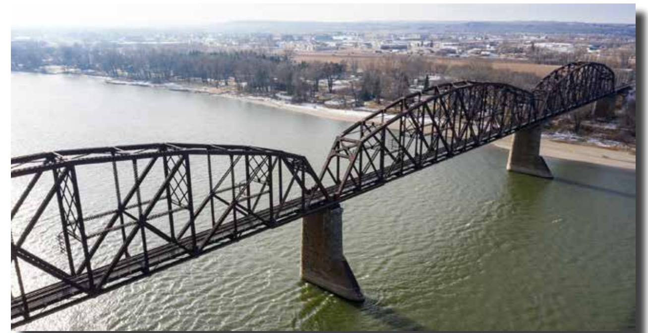
[figure 1.1] aerial drone view of high bridge
