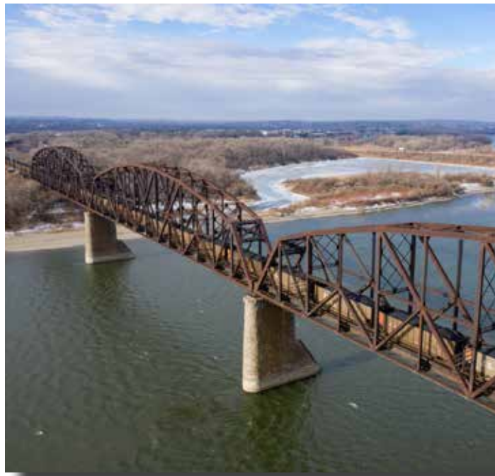
figure 1.0] aerial drone view of high bridge
